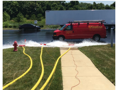
Fire Pump Test on a Sunny Day
