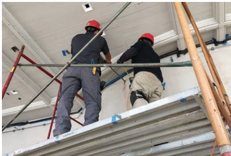
Installing a Water Mist System in a Historic Museum
