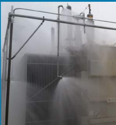
Acceptance Test on a deluge system that we just installed at BGE Finksburg
