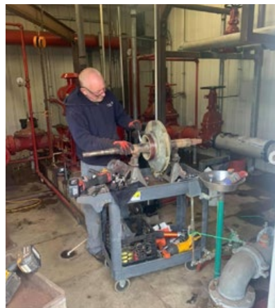
Tim Gott Rebuilding A Fire Pump
