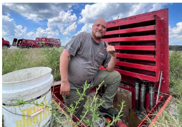
Flushing underground vault hydrants at BWI
