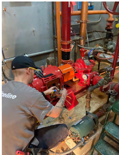
Fire pump rebuild
