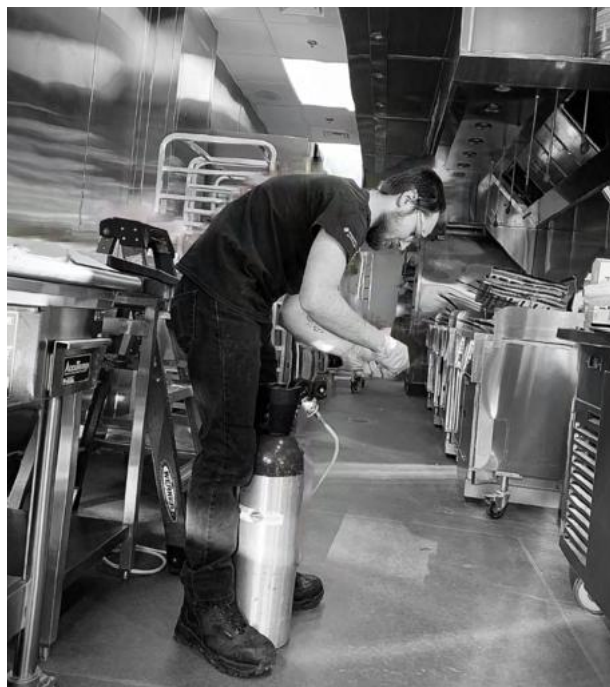
Joe Parmer working on an install
