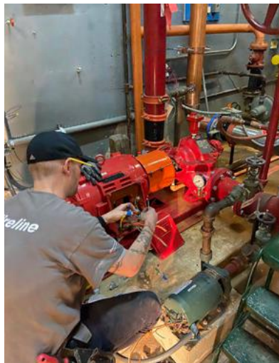
Fire pump rebuild
