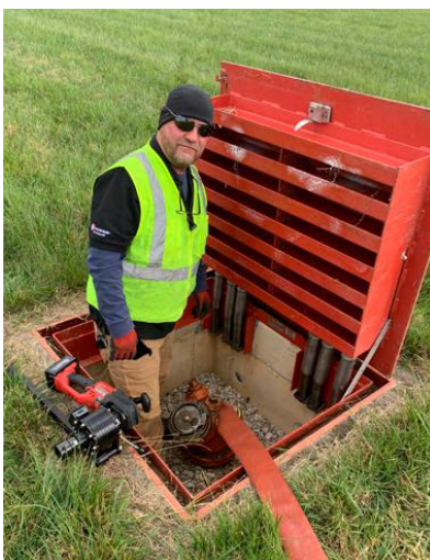
Hydrant testing at BWI
