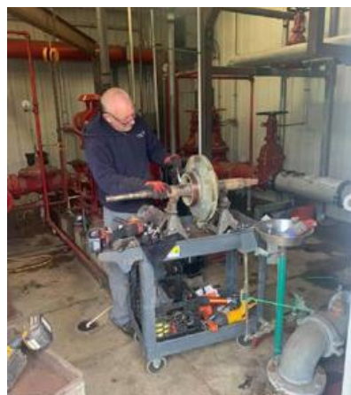
Tim Gott Rebuilding A Fire Pump
