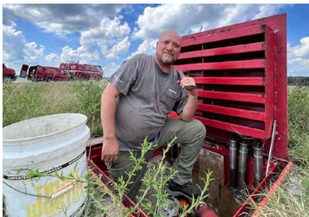
Flushing underground vault hydrants at BWI
